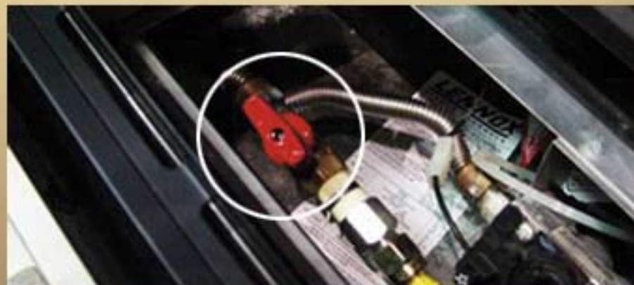
Gas supply in the ON position
